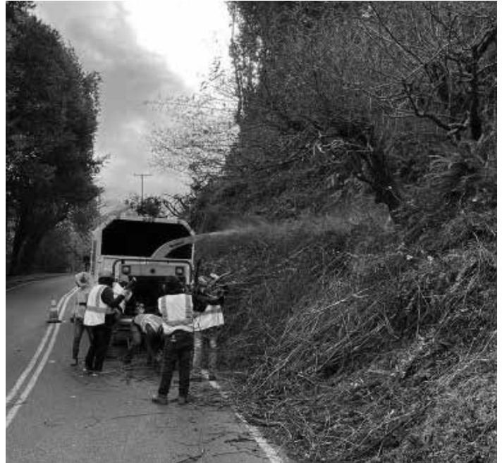
Brush and tree removal and chipping in-progress.
