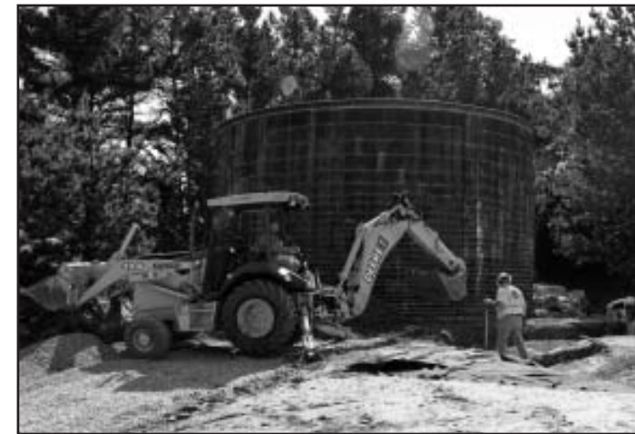
Huge backhoes removed tons of soil and boulders from the berm bordering the Overlook and piled it temporarily on top of the existing berm along Seacape. Here, the new tank's foundation is being roughed out.
