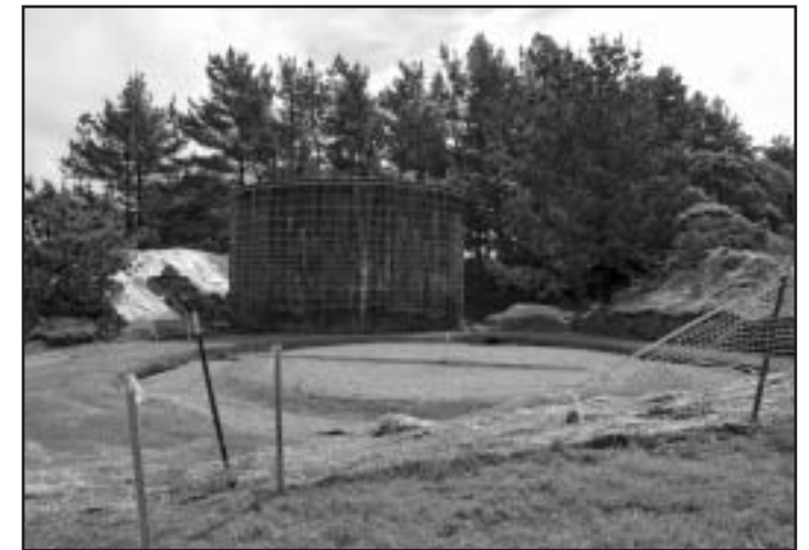
This photo was taken from approximately the same place as the "Before picture." The gravel bed has been placed, leveled and compacted, ready for the tank to be built beginning in early April. The earthmovers will return in June to re-configure the area surrounding the tanks. When finished, the new tank will be partially buried and concealed by a new berm and landscaping.
