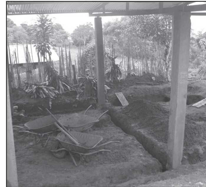
Chirapa School kitchen construction project. We excavated and raised the columns and put up the roof. Work will continue on footings and walls.
