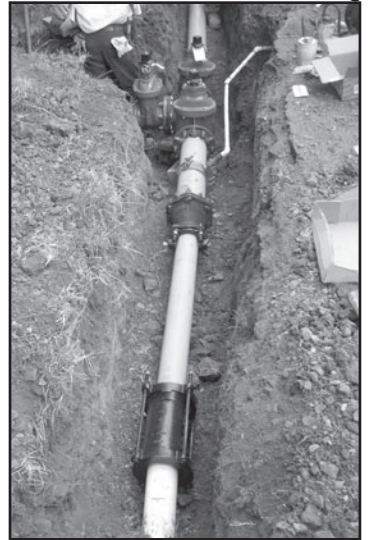
View of new pipe connecting Sunset Way service line to the water main along Highway One, near the entrance on Sunset Way. Note this is all buried under Sunset Way and paved over, albeit with access to the shut off valves.
