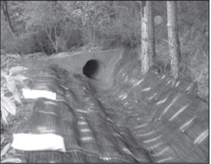
Bello-Seacape drainage ditch and culvert
